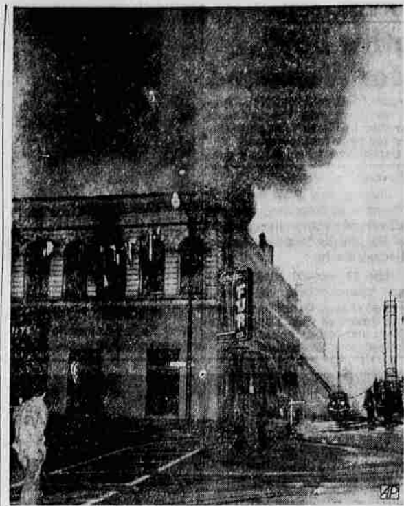
Firemen Fight Hotel Blaze—Smoke billows from Lafayette Hotel at Aberdeen, Wash., as firemen (right) direct streams of water on the blaze that caused seven deaths. Hotel rooms were on second floor, with shops on street level. (AP Wire-photo)
