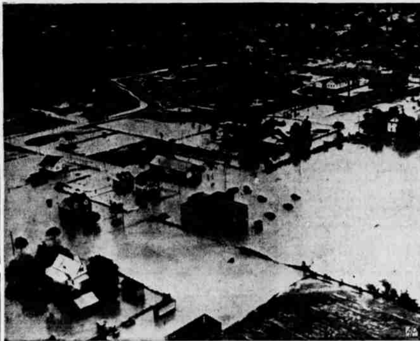
Flash Flood General View—This is a general view of the outskirts of Moorefield, W. Va., after a flash flood inundated a good portion of the community. Stranded autos can be seen surrounding the large building in lower center. More than a dozen persons reported missing. State Police Capt. Basil E. Wright said at Elkins, W. Va., that indications were that many hundreds were made temporarily homeless and that property damage was heavy. (AP Wirephoto)
