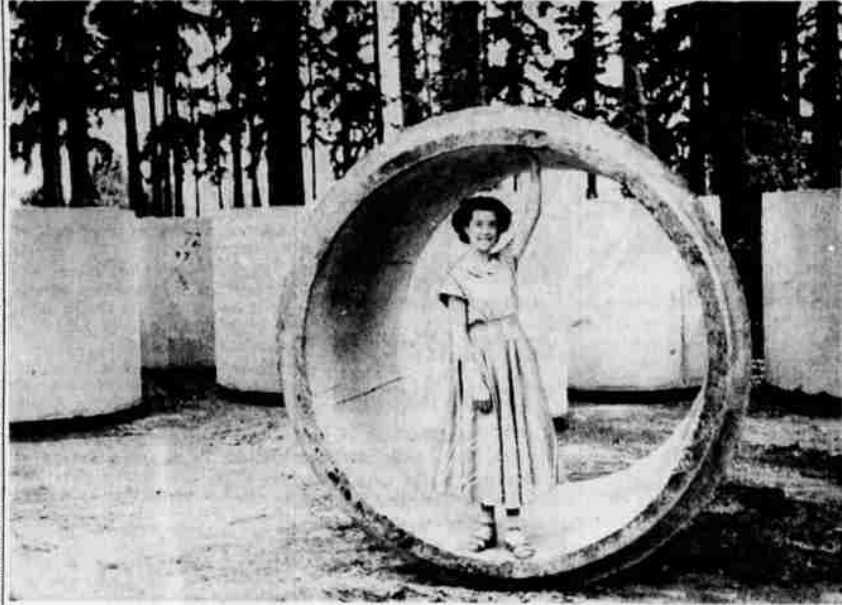
Big Enough for Housekeeping—Loretta Sizemore, 345 Hickory street, who is five feet and three inches in height stands comfortably in a 72-inch section of pipe now being manufactured in Salem by the Seattle Concrete Pipe company for use in an interceptor sewer to extend from the river to Church and Union streets. Each section contains three yards of concrete, is reinforced with 300 pounds of wire mesh and weighs six tons. Three pipe sizes, 72, 66 and 60 inch are being manufactured for the line approximately 11,000 feet in length. Laying to a depth of 27 feet will begin sometime in June.
