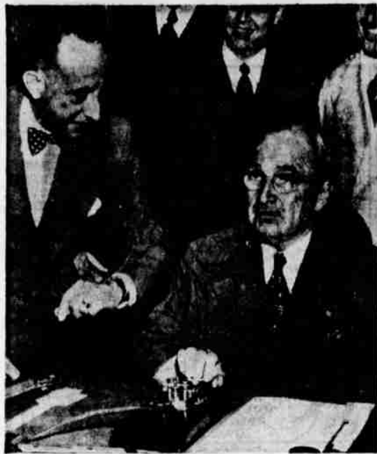
Electrifying Event —White House aide Russell McMullin gives President Truman a time check as the president presses a gold key in Washington, D. C., giving the signal to put the 10th main generator at Grand Coulee Dam, Wash., into commercial operation. The president hailed the event as one more step in harnessing the almost limitless power potential of our great northwest. (Acme Telephoto)
