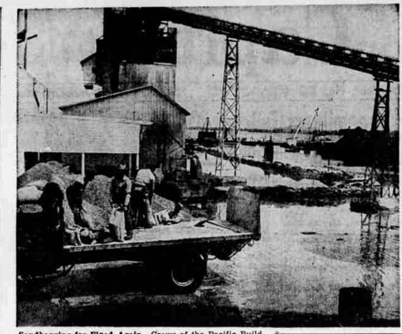
Sandbagging for Flood Again—Crews of the Pacific Building Materials company at Vancouver are kept busy supplying bagged sand for flood wary districts along the Columbia river lowlands. Some industries stock-piled for emergency use. (AP photo)
