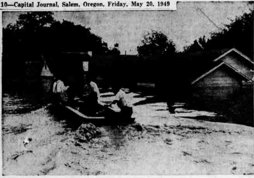
Flood Victims Inspect Damage —Victims of the sudden flood which surged into West Fort Worth, Tex., ride down the street, or about eight feet above, to inspect the damage done to their inundated homes. The flood was the result of a 10-inch deluge of rain which sent the Trinity river smashing through four levees into an estimated 100 square miles of the city's metropolitan area. The weather bureau forecast more thunder showers for the area, which would send the slowly falling river still higher. (Acme Telephoto)
