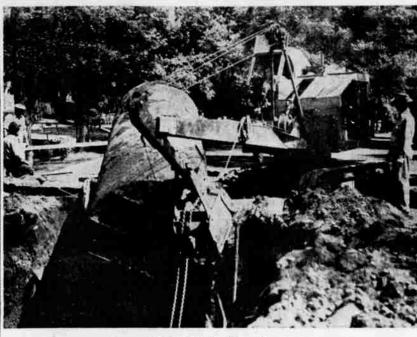
heating plant for the old capitol was converted from wood to oil 35 years ago this 15,000 gallon tank weighing near five tons was used for fuel storage. E. J. Slick, Salem excavator, now digging for an access tunnel between the new state office building and the capitol, removed the bulky tank with his small Bucyrus-Eric shovel though not at the first attempt.
