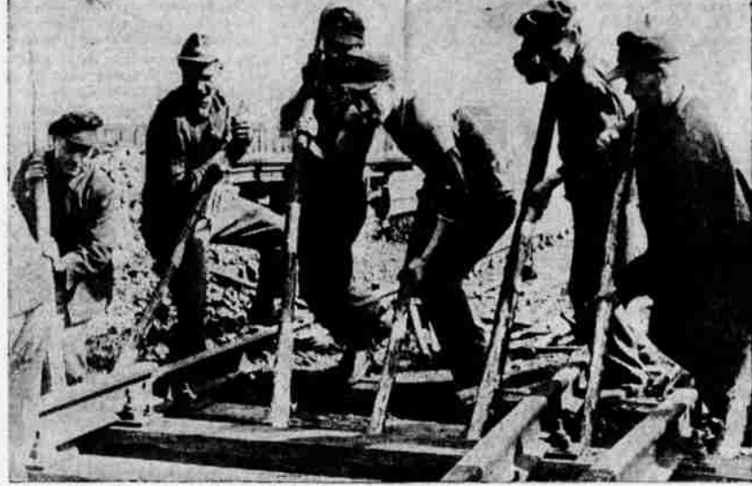
Rails Repaired as Blockade Ends—As Big Four powers agree to lifting of Berlin blockade, German railroad workers repair switch-rails at the Grunewald station in the British sector of Berlin...
