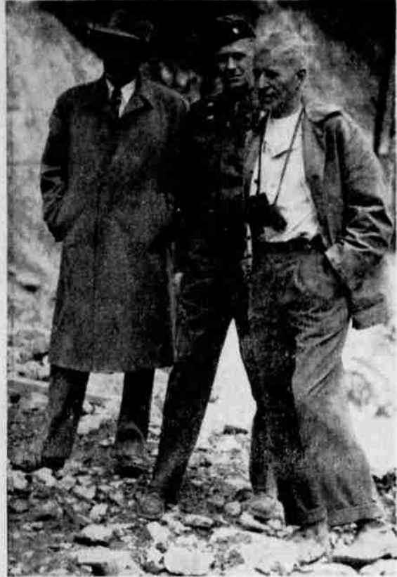
Inspecting the Detroit Dam Site—Three key figures in construction of the Detroit dam on the North Santiam river are (left to right): T. M. Price, expert on aggregates; Lt. Col. J. W. Miles, resident engineer of Corps of Engineers; and Russell Hoffman, superintendent of the job for Consolidated Builders. They are shown overlooking the lowering of coffer dams at the construction site.
