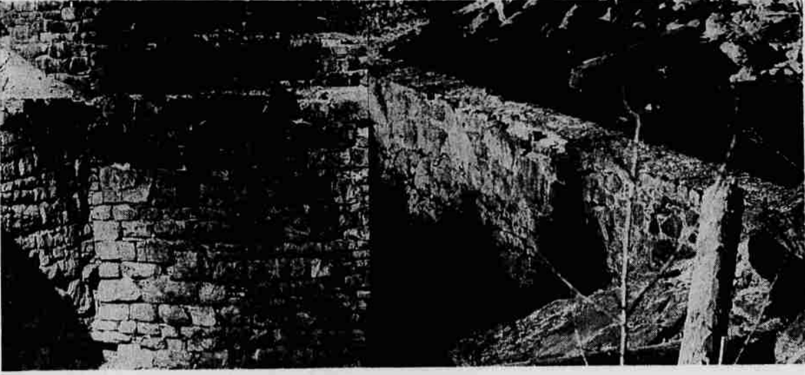
Weathered Masonry, Relic of Niagara's Thwarted Progress— Left: Beautifully cut and laid stone placed by O'Neil brothers about 1900 to control and divert waters of the North Santiam through a hydro-electric power project. It now looks like some fragment of an ancient ruin. Right: Masonry dam, another part of the $100,000 project developed over 25 years but without any worthwhile accomplishment.
