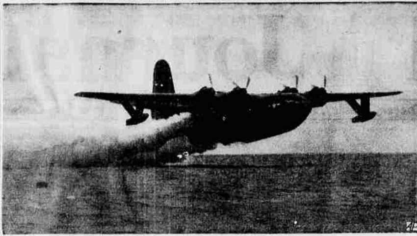
Mars in Jet-assisted Takeoff (JATO)—Using twelve rockets in relays as an assist in the takeoff, the navy's flying boat Philippine Mars (above) was airborne in a test flight at Alameda, Calif., in about 40 percent of the time usually required. During test the Mars weighed 70 gross tons.
