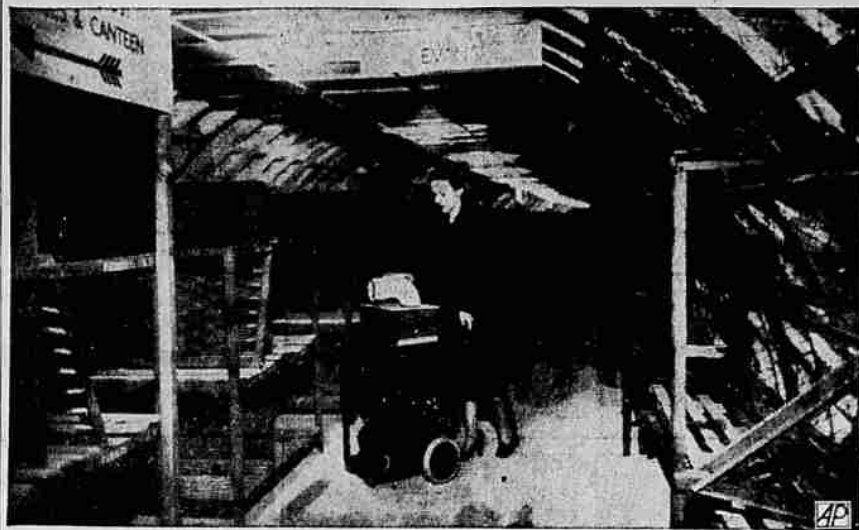
Huge New London Raid Shelter Prepared for Occupancy—An air raid precaution worker operated a vacuum cleaner type of apparatus in cleaning one of London's huge, new deep-tunnel air raid shelters, built far below the ground and beneath subway stations. Each shelter is capable of sheltering 8,500 persons. Tiers of bunks stretch as far as the eye can see. There are to be eight such super shelters, seven of which were expected to be ready this fall in event of reopening of air attacks on the city. — Associated Press Photo.
