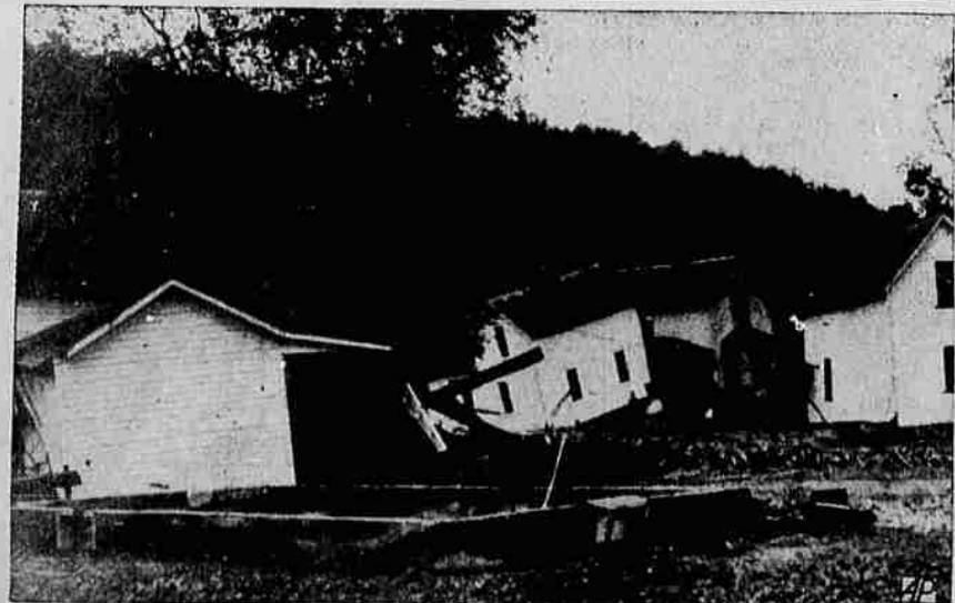
House Moved by Flash-Flood—Leaving the foundation intact, a house was moved 150 feet to come to rest on a neighbor's porch (center foreground), when a flash-flood swept through Spring Valley, Wis. No lives were lost in the flood. All of the residents found refuge in nearby hills. (Associated Press photo.)
