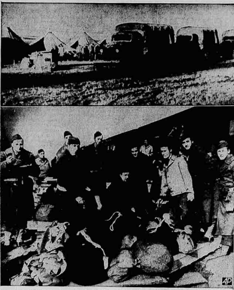
U. S. Army Camp Set Up for Alaska Road Job—A U. S. army camp (top), has been established seven miles from the end of the railway at Dawson Creek, B.C., for the start of work on the highway to Alaska. Below: U. S. soldiers, who will help build the highway, have their luggage piled high on the station platform at Dawson Creek. One at left had a hasty snack. — Associated Press Photo.
