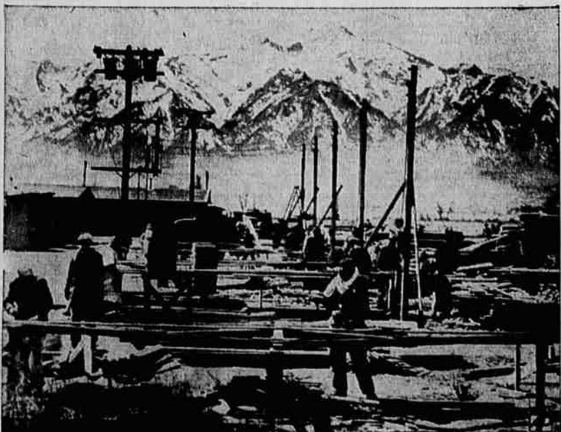
Work Speeded on Japanese Evacuation Center—With the snow-capped peaks of the Sierra Nevada towering in the background, workmen rushed construction on the huge reception center at Manzanar, Calif., in Owens valley, to prepare it for the reception of the first of 10,000 Japanese to be evacuated from southern California. Lieut. Gen. John L. DeWitt of the western defense command, commandeered 6,000 acres for the boom town. — Associated Press Photo.
