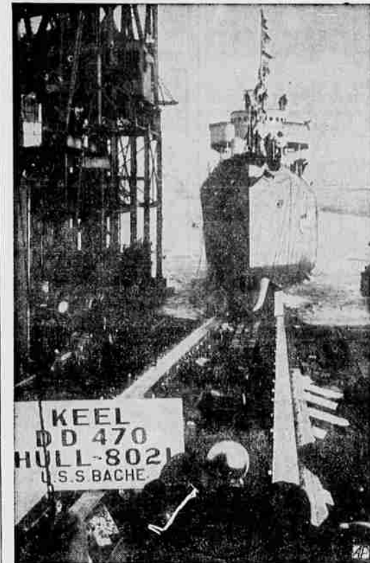
Destroyer Assembly Line—As the U. S. destroyer Farenholt, a sister ship of the torpedoed Kearny, was launched at the Bethlehem Steel company's State Island, N.Y., shipyard, work started on the same ways on the keel of the U.S.S. Bache, another destroyer. — Associated Press Photo.
