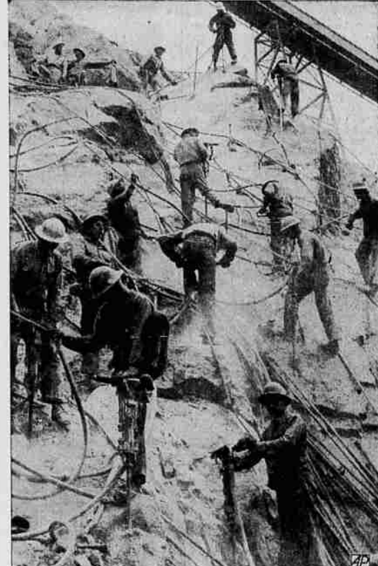
Drillers Work On Shasta Dam—Jackhammer men are drilling dynamite holes to blast out rock high up on the wall of the Sacramento river canyon for the west abutment of Shasta dam. They are operating drills powered by compressed air which is conveyed to all parts of the construction area by steel pipe and rubber hose from a central compressor plant. — Associated Press Photo.
