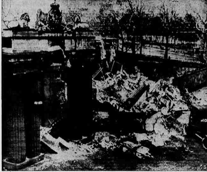
Buckingham Palace Lodge Bombed—An air raid bomb caused this damage at a Buckingham palace lodge at London recently, wrecking the lodge house and part of the pillars of the portico at the left. This cable photo from London shows the Royal insignia still surmounts the pillars. — Associated Press Photo.
