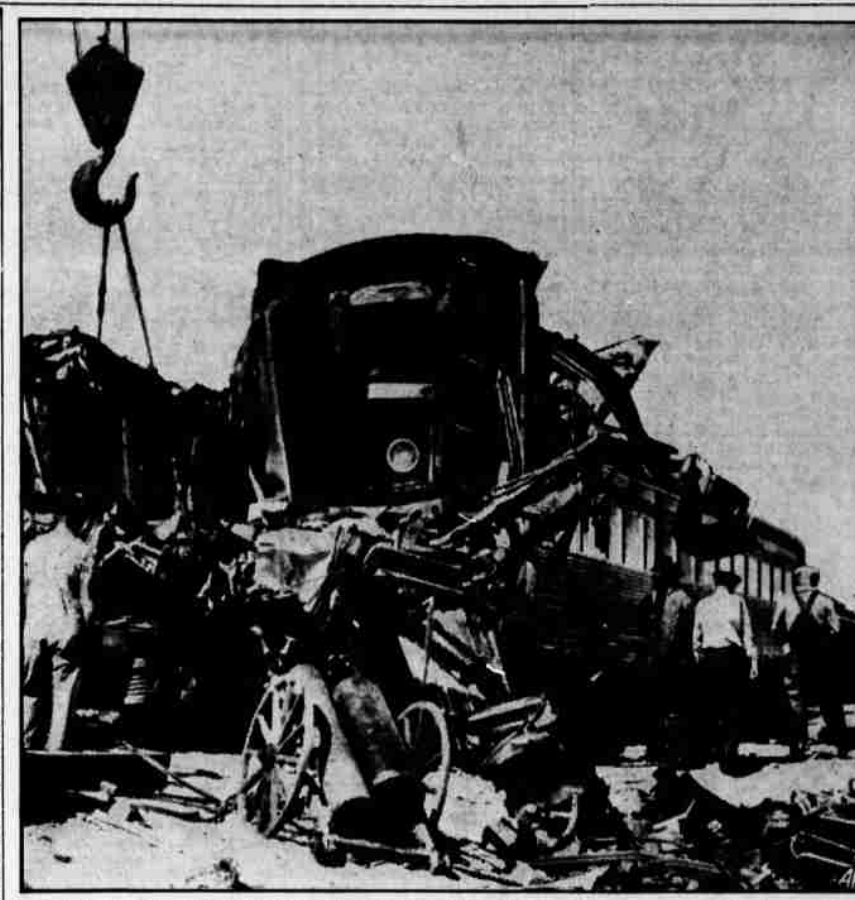
Passenger Trains Collide Head-On; Eleven Killed—Streamlined coaches were crushed in the terrific collision of two crack Southern Pacific passenger trains on a siding near Niland, Calif., and eleven persons were killed and 100 injured, some critically. The streamlined coach (above), shows how the impact crumpled it. A brakeman's mistake was blamed for the tragedy. — Associated Press Photo.
