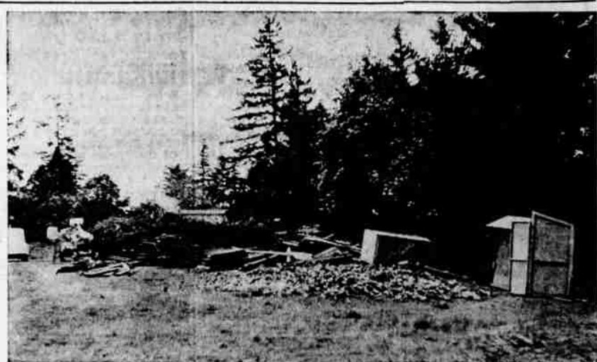
Residents of Fairmont Heights contemplate the above pictured storage yard for surplus and unused construction materials and equipment of the city water department on the site of the old reservoir with violent resentment. A sample of the ornaments with which the dump is being adorned is the portable "Chic Sales" edifice of pea-green hue pictured below.
