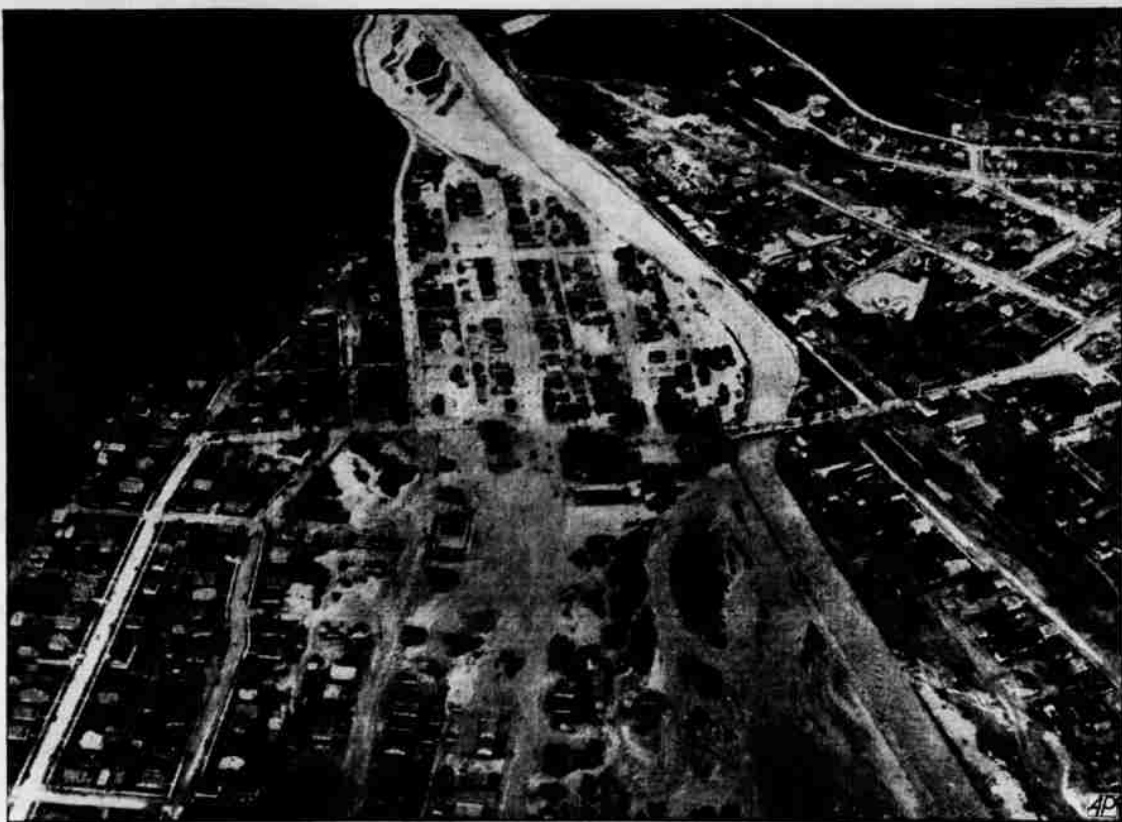
Wild River Floods North Idaho Town—Many residents of Kellogg, Idaho, were driven from their homes by flood waters of the south fork of the Coeur d'Alene river, which went over its banks after three days of snow-melting rains. This airview shows how the river cut a swath through the town. It was made by the 118th photo section, Washington National guard. — Associated Press Photo.
