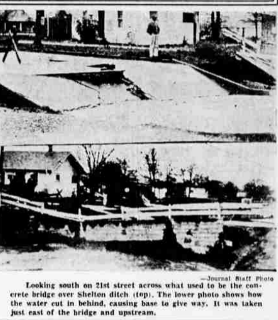
Looking south on 21st street across what used to be the concrete bridge over Shelton ditch (top). The lower photo shows how the water cut in behind, causing base to give way. It was taken just east of the bridge and upstream.
