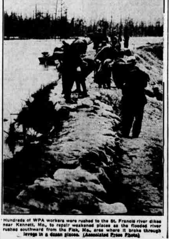
Hundreds of WPA workers were rushed to the St. Francis river levee near Kennett, Mo., to repair weakened places as the flooded river rushes southward from the Flak, Mo., area where it broke through levee in a dam place. (Associated Press Photo)
