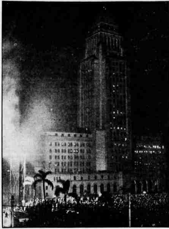
This picture shows the burst of brilliant light that resulted when the first power from Boulder Dam project, 266 miles away, reached Los Angeles. Its arrival was heralded with the lighting of a huge electric arc which cast its light on the buildings of the Civic Center. The arc is at the left, with the city hall in the background. (Associated Press Photo.)
