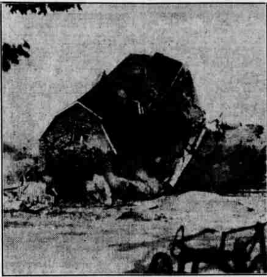
The camera clicked as this house tumbled to earth just after 60 pounds of dynamite had been discharged. The two-story structure, a former life-guard house, was destroyed to make way for a new boardwalk at a New York beach. (Associated Press Photo)
