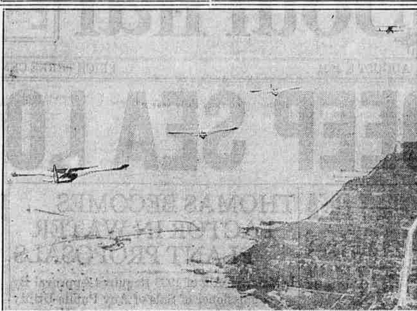
Here is an airview of the "sky train" of gliders that left Floyd Bennett field, Brooklyn, N. Y., carrying mail to Philadelphia, Baltimore and Washington. Fastened together behind a "locomotive" biplane, the three gliders are shown riding gracefully a short time after the takeoff. A few hours later the train landed at Philadelphia, the three gliders being detached to ride to a graceful landing. Storm conditions there forced a halt in the flight until the following day. (Associated Press Photo)
