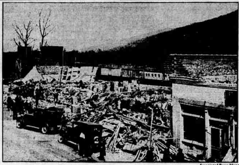
Four persons were killed when a hosiery mill in Paint Rock, Ala., was struck by one of the tornadoes which caused widespread damage and loss of life in the south. The ruins of the mill are shown above.
