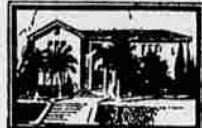
Electro-Kold equipped home of Vincent Palmer, Los Angeles.
