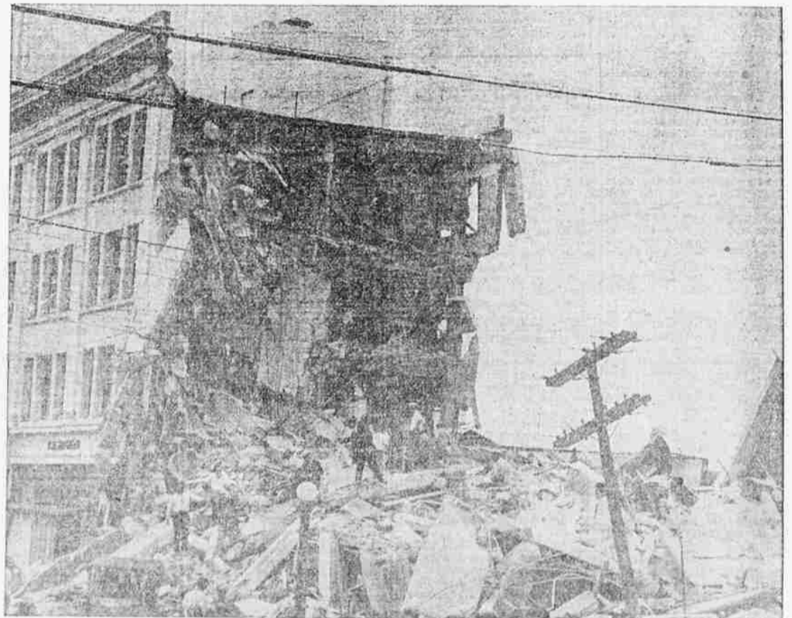
What was left of the San Marcos Building, the largest business structure in Santa Barbara after the earthquake of June 29. Copyright, 1925, by International Newsreel.
