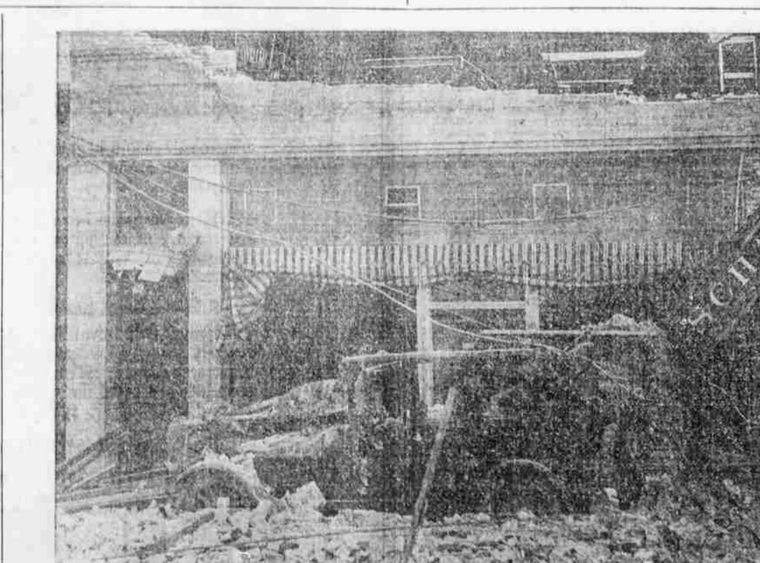
View of Santa Barbara Garage after Earthquake. Two are believed to have been killed when this structure collapsed. Copyright, 1925, by International Newsreel.
