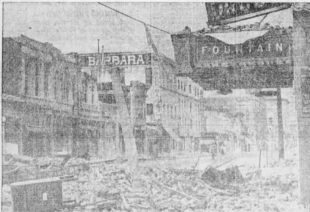
Havoc wrought on State street, Santa Barbara by the June 29 earthquake. Practically every building on this street was damaged. Copyright, 1925, by International Newsreel.
