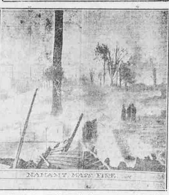
A terrific blaze swept through the Summer colony at Nahant, Mass., and destroyed thirty-five cottages with a damage of $250,000. Scores were made homeless by the fire which was finally checked by fire departments assembled from six cities.
