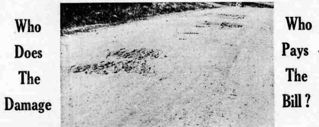
Section of Pavement Between McMinnville and Sheridan
