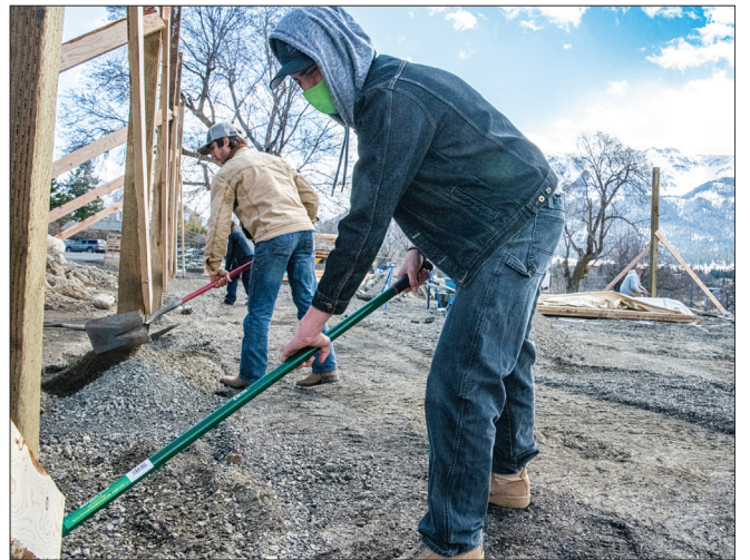
Ellen Morris Bishop/For the Wallowa County Chieftain Joseph Charter School agriculture students Laramie Hass, right, and Trace Collins fill in gravel around the newly set uprights for a new "bull barn" on the northwest end of school's campus. The structure, funded by an Oregon Department of Education revitalization grant, will provide a better shelter for student ag and FFA livestock, including pigs, said JCS ag teacher Chelcee Mansfield.
