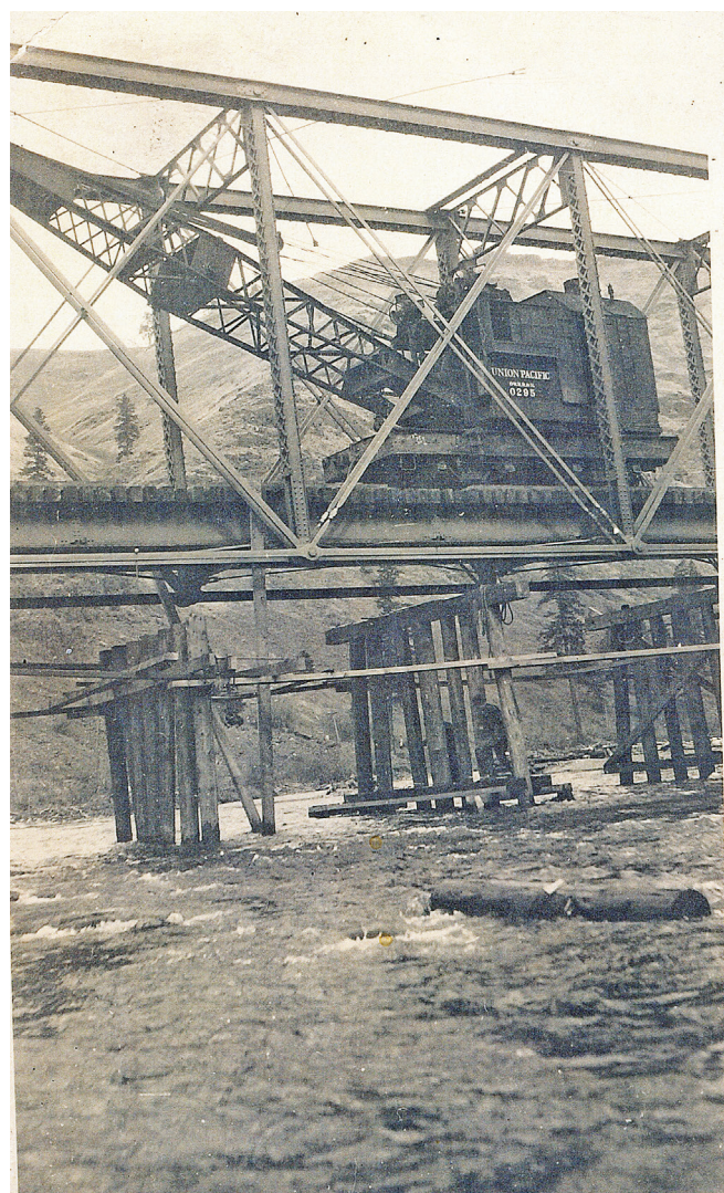
Bridge repair, Wallowa River at Minam. Photo courtesy of Edsel White.
