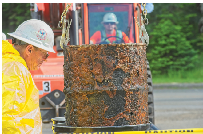
Photos by Ellen Morris Bishop A member of the hazardous materials crew watches as a rusted barrel is lifted from its containment "overpack" for inspection and testing June 15.
