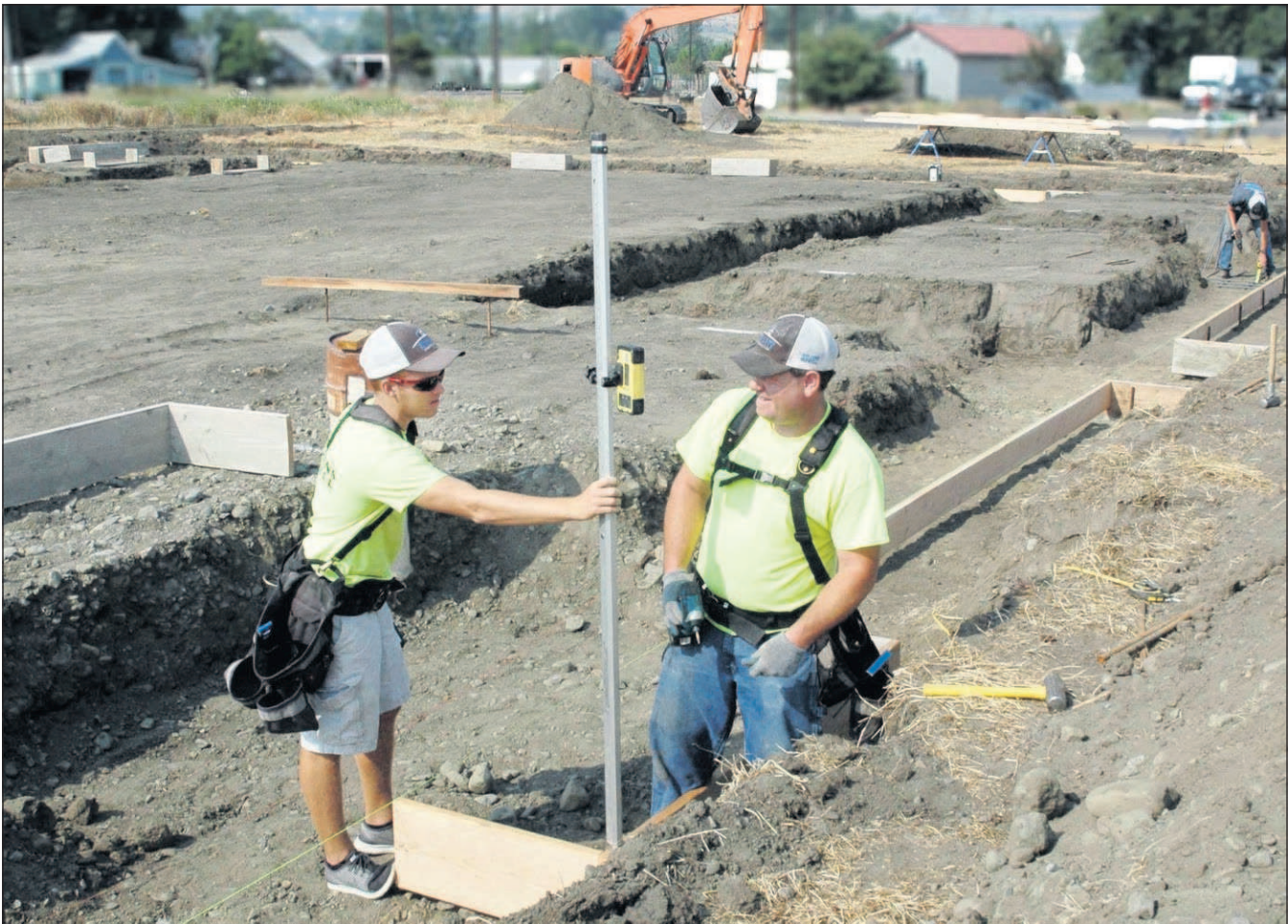
Kathleen Ellyn/Chieftain Karl Wellens of Wallowa and Jason Yarborough of Lostine work in the footings of the new 10,000 square-foot Enterprise Electric building. It will be the first energy net zero building in the county.
