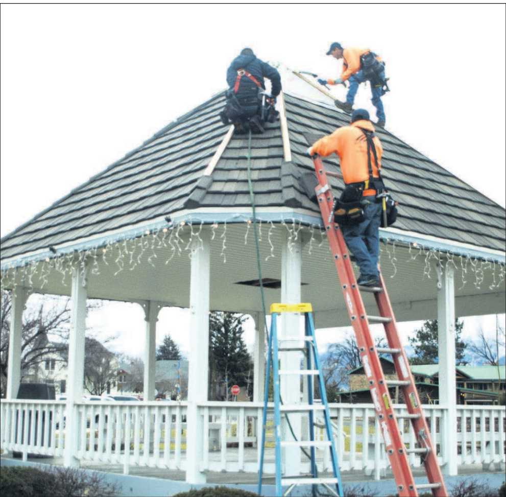
Photo courtesy of Rotary Club of Wallowa County Palmer Roofing Co.'s crew places the last of the roofing on the Courthouse Gazebo.
