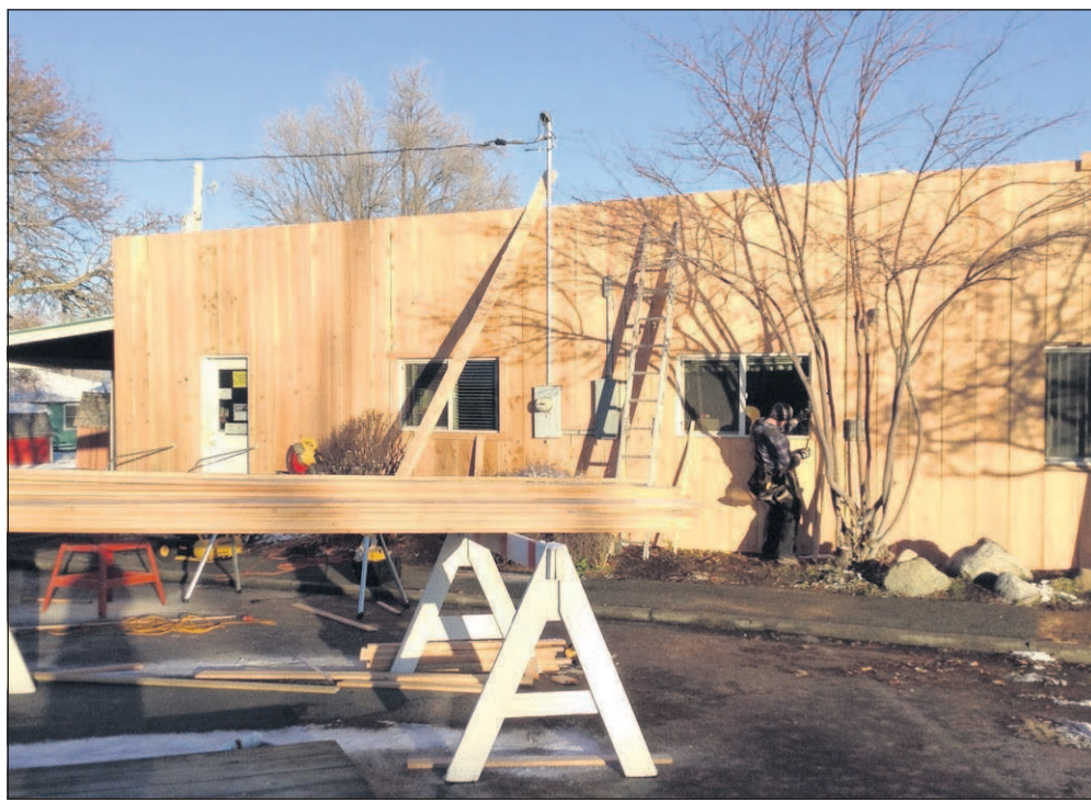
Joe Vinni places new siding on the Joseph City Hall building.
