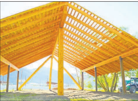
Steve Tool/Chieftain This photo from mid-July shows nearly completed roof of the new arbor at the rodeo grounds in Joseph. Shingles were added to the roof prior to Chief Joseph Days.
