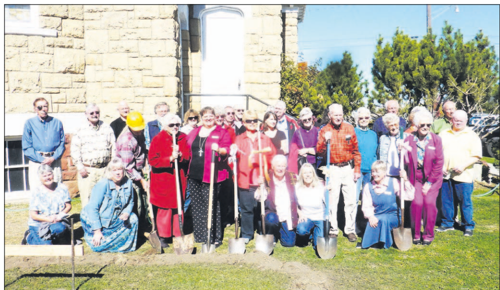
The congregation of Joseph United Methodist Church stand next to the foundation of their new Fellowship Center. After posing for photos, the group broke into an impromptu version of the gospel standard "Holy Ground."
