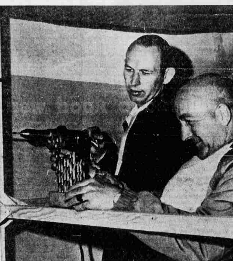
LIONS BOSSES—Generally supervising work this morning when Lions constructed booths for their three day Home Show starting Thursday evening at the Armory were these two men. At left is Will M. Storey, using electric equipment, and at right is Maurice Shelton, general chairman, with booth plans under chin and drill in hand.
