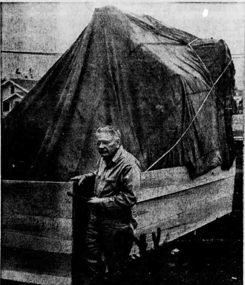
EMERGENCY POWER —Lee Reinhart, maintenance engineer for St. Charles Memorial hospital, touches up the board protective wall around a surplus government 100 KW generator. The present generator has a capacity of 15 KW which supplies power to the delivery rooms, surgery, and several other important areas. The new power plant when installed this summer should supply power for the entire hospital in case of an electrical shortage. Brooks-Scanlon and Bend Redi-Mix furnished heavy equipment and men for unloading the power plant.
