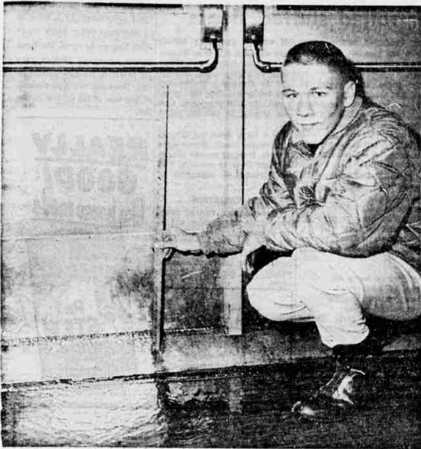
"—AND RISING"—Afternoon downpour Wednesday sent flow of water under doors of Wing C's east entrance at Bend High School. Mike Murphy, with yardstick, made like the weatherman. Students hopeful of early start for Christmas vacation were disappointed. Water receded after storm, and classes were in session as usual this morning.
