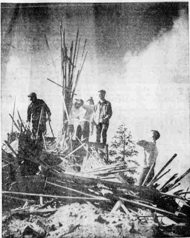
BUILDING BON FIRE — Boys from Bend High school worked hard most of the day Friday building a huge bonfire for Homecoming. Unloading lumber from a truck at the old Ryan field are from left to right Kerry Yancey, Jake Young, Frank Nicholson, Glen Rea (hidden behind Nicholson), Dean Seers, and Ken Collier.
