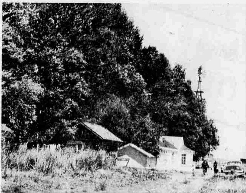
"THE POPLARS" — One of Central Oregon's best known ranches is "The Poplars," home of Mr. and Mrs. Bud Parks, at Fort Rock. This is a summer view of the Parks' home. Visible above the trees, but now a bit out of date, is a windmill. Water is now pumped electrically. (Bulletin Photo)
