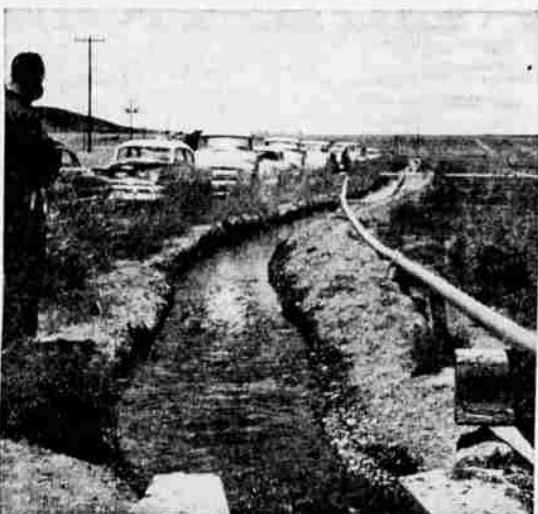
LIFE OF THE LAND — This stream, flush with water needed for the irrigation of Fort Rock land, is pumped to the surface by use of electricity. Both flood and sprinkler irrigation are in use.
