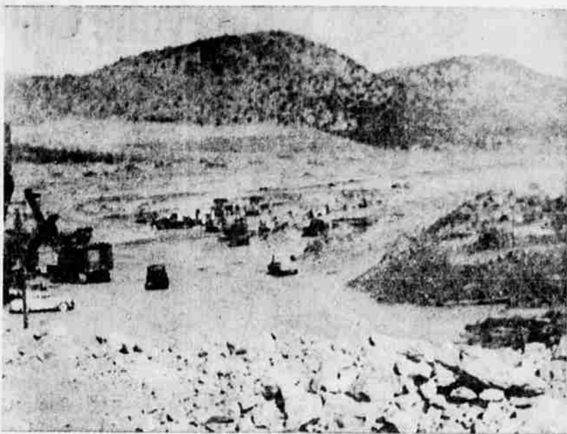
VIEW OF BASIN FROM DAM'S TOP — Broken rock in the foreground is at the top of Haystack dam, 80 feet above the low point of the upward sloping reservoir in the center of the picture. It is surrounded on three sides by hills in the background. (Bend Bulletin Photo)
