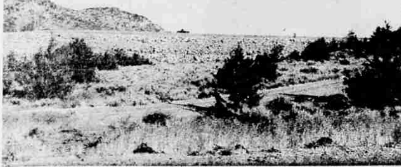
FRONT VIEW OF HAYSTACK DAM — This photo was taken of the 80 foot high Haystack dam of dirt and broken rock at a distance of 200 yards. The dam will hold water to be stored in a large basin on the other side. (Bend Bulletin Photo)
