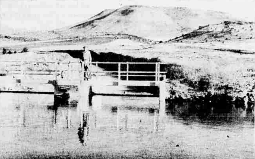
TURNOUT STRUCTURE — Water from the main canal (shown in foreground) will be sent through this turnout structure into the feeder canal beyond which will take it into the two billion gallon capacity reservoir. (Bend Bulletin Photo)
