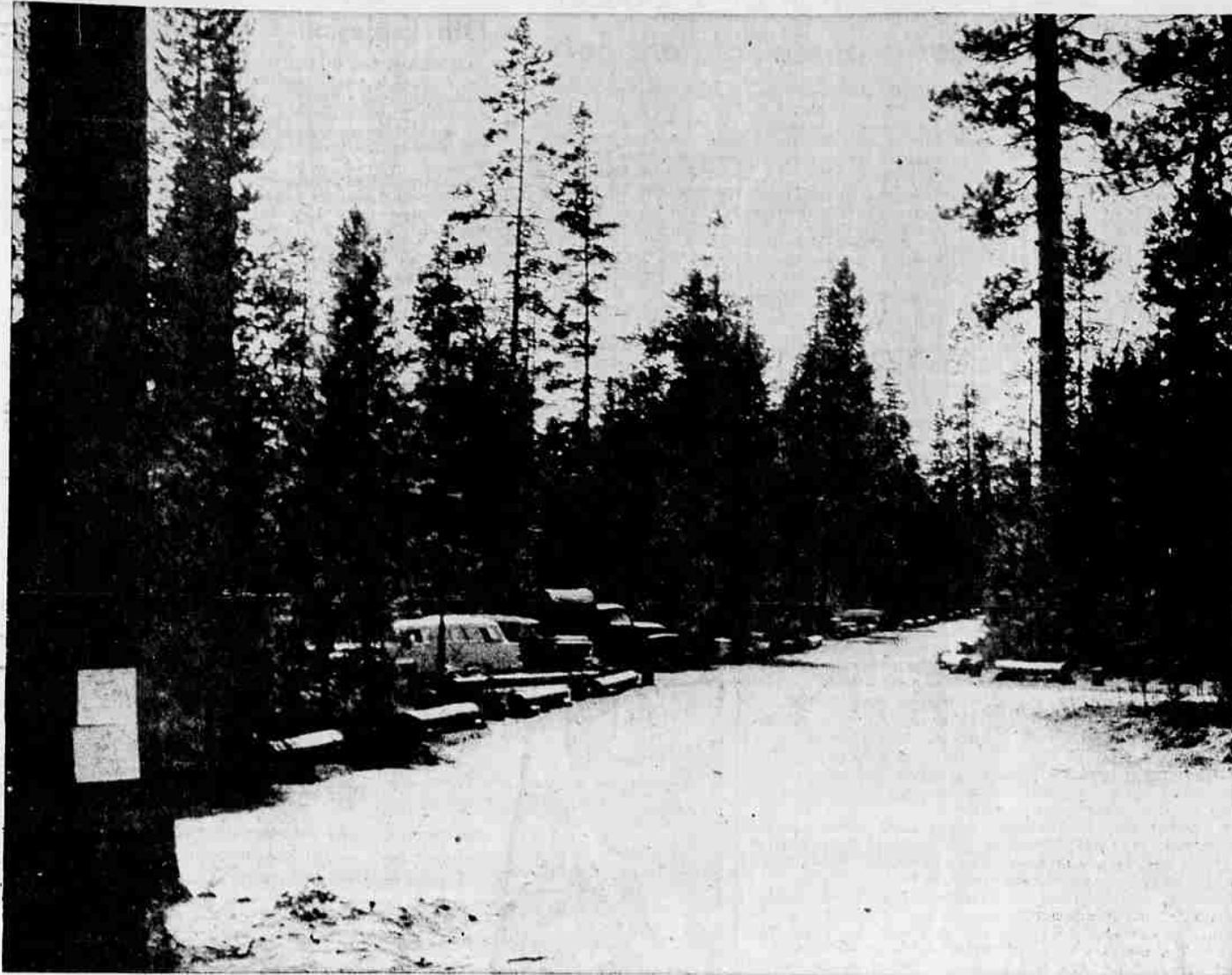
NEW CAMPSITE TAKES SHAPE IN DESCHUTES FOREST This is a view west along the new camping loop at Wickiup Reservoir area
