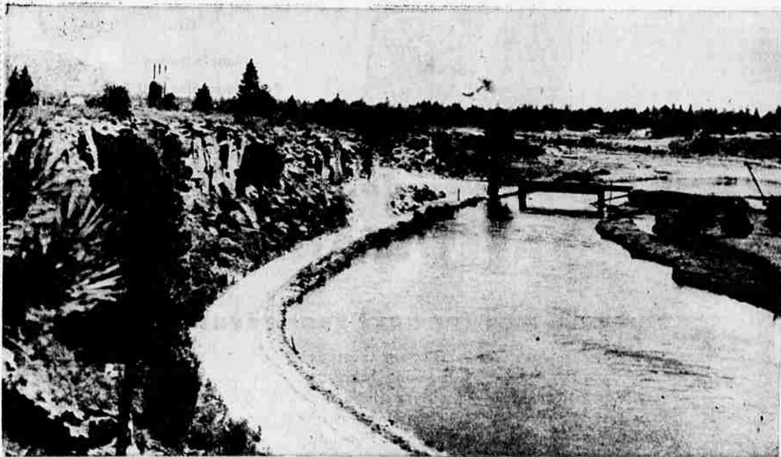
NEW SPAN TAKES SHAPE OVER DESCHUTES RIVER View, downstream, shows Brooks-Scanlon logging road bridge
