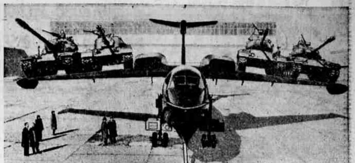
IT HAS HEAVY "WING TANKS"—No, those tanks weren't really atop the wings of this XP6M-1 Martin Seamaster. It's a composite picture, fixed up to dramatize the amount of stress the wings can take. The Navy's new multijet seaplane, to be flight-tested this spring, is undergoing a series of rigorous structural tests in its Baltimore, Md., hangar. Wings alone have been subjected to an applied load of approximately 350,000 pounds, which is about what the tanks represent.
