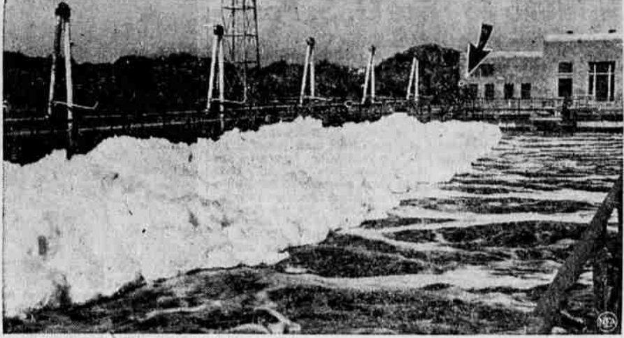
IT ALL COMES OUT IN THE WASH —When mama does the family washing with some of today's free-sudsing detergents, employees of the Canton, Ohio, sewage disposal plant see the results a few hours later. This picture shows the foam that collects in just one of the aeration tanks at the plant. One man (arrow) has practically a full-time job attempting to wash away the tidal wave of suds with a hose.
