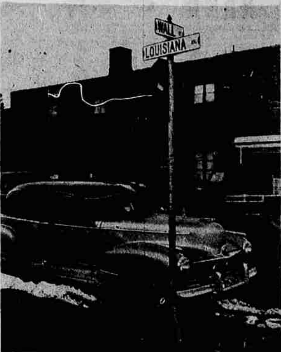
New street signs, of steel with baked enamel facing, now are being put up in Bend by city street department crews. The city has purchased 151 of the new signs. Estimated cost of the signs, plus installation, is $2,000.
