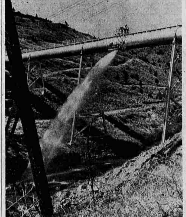
Farm tourists on their swing through the North Unit of Jefferson county earlier this week were given a demonstration of the manner the huge siphon that carries Deschutes water across Willow creek, near Madras, is drained. When a vent was momentarily opened, a great stream of water sprayed into the Willow creek gorge. The siphon carries 500 second feet of water to the Agency Plains lands.
