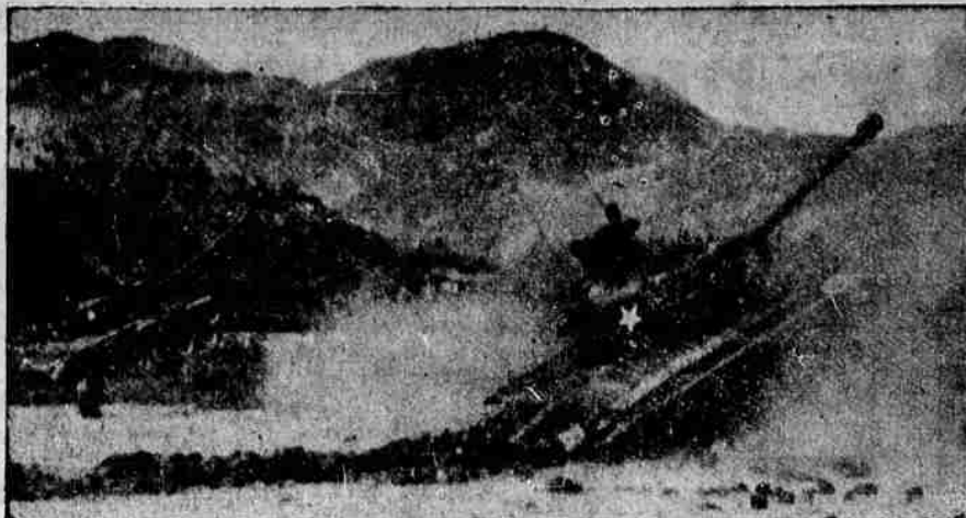
TANKS DIG FOR DISTANCE —Their front ends jacked up on mounds of earth piled high by a tank mounting a bulldozer blade, these two armored giants fire their guns in support of U. S. ground troops fighting west of Masan, South Korea. The dirt mounds act as platforms to raise the gun barrels, giving the shells much greater range.
